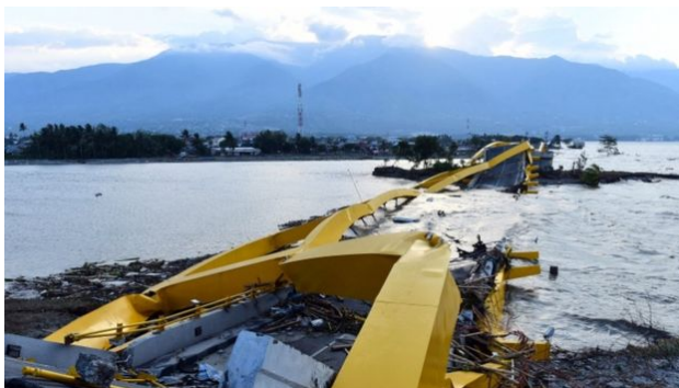
A bridge was destroyed by the tsunami
